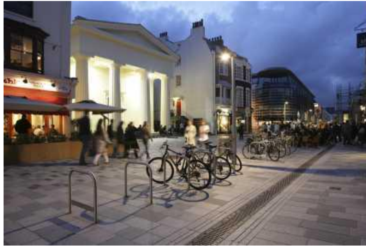
Picture: Shared surface road in Brighton: an essential component of traffic calming
