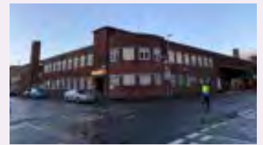
Bus offices and garage building with its distinct 1930's architecture
