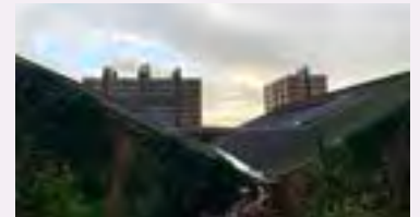
The 10 storey residential tower blocks form prominent elements within the townscape to the south of the station
