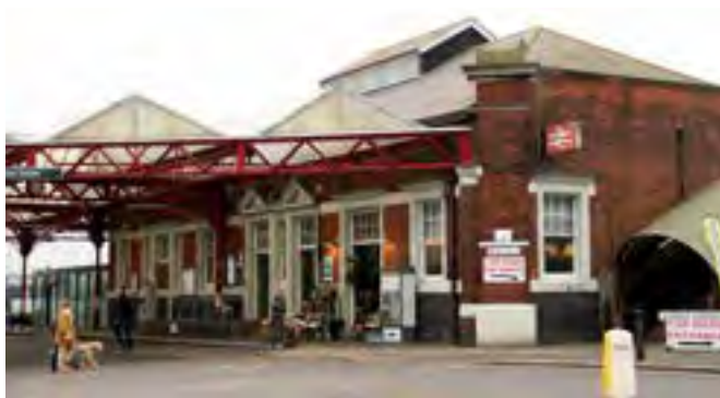
Above - Figure 3.7: Hove Railway Station and footbridge
